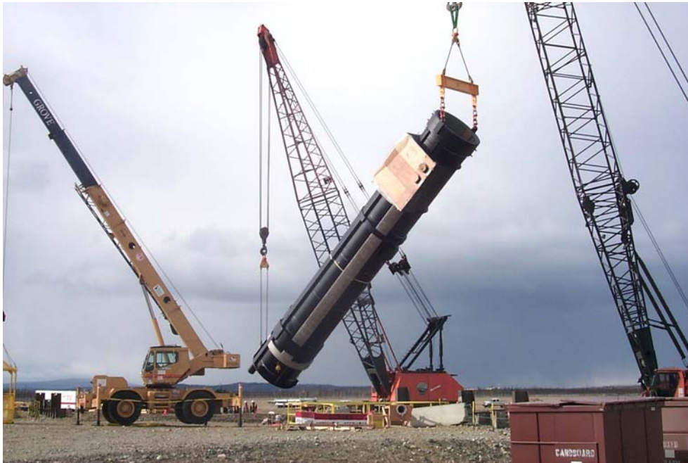
Fig. 6-20. Installation of the first of six Ground-based Midcourse Defense missile silos at the GMD Testbed at Fort Greely, Alaska in 2003. The 75-foot long silo weighs 130,000 pounds.
